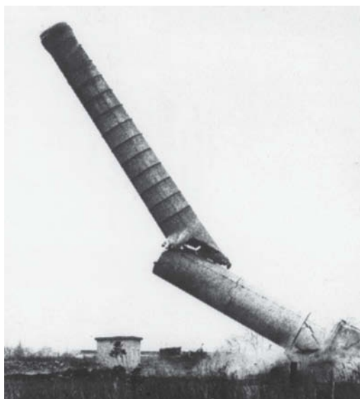
FIGURE 8-9. A falling chimney often is not strong enough to provide the tangential acceleration at large radius that is necessary if the entire object is to rotate like a rigid body with constant angular acceleration. See “More on the Falling Chimney,” by A. A. Bartlett, The Physics Teacher , September 1976, p. 351, for an account of this phenomenon.
